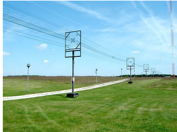
A type of transmission line called a cage line, used for high power, low frequency applications. It functions similarly to a large coaxial cable. This example is the antenna feedline for a longwave radio transmitter in Poland, which operates at a frequency of 225 kHz and a power of 1200 kW.
